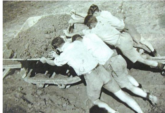
The boys building the North Sea Camp.
