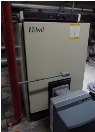
One of two floor standing boilers used for the main heating of the school
