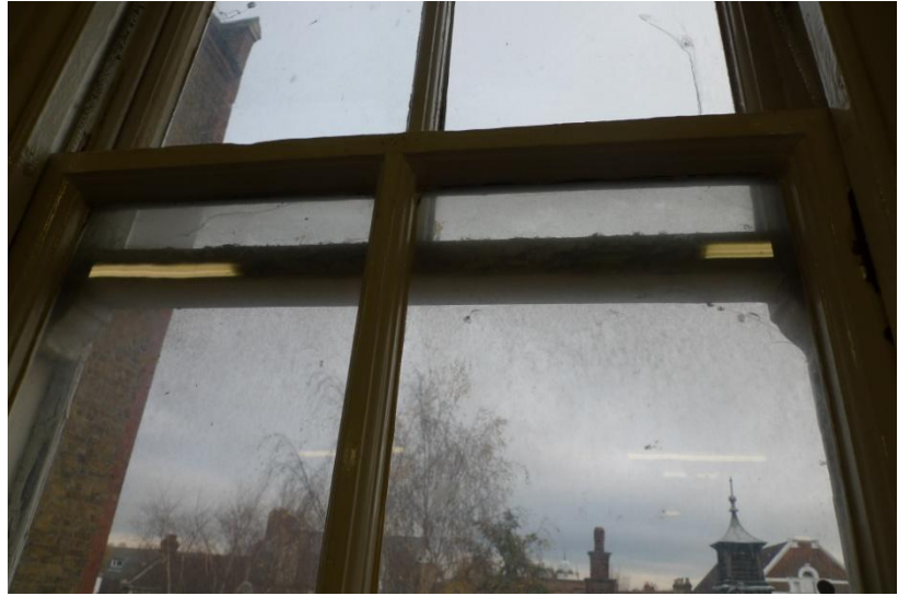
Several of the original sash windows don't fully close
